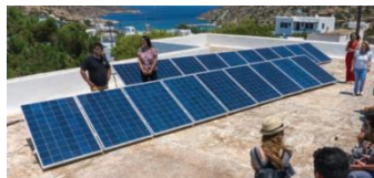
Installation of a PV system on a high school roof
