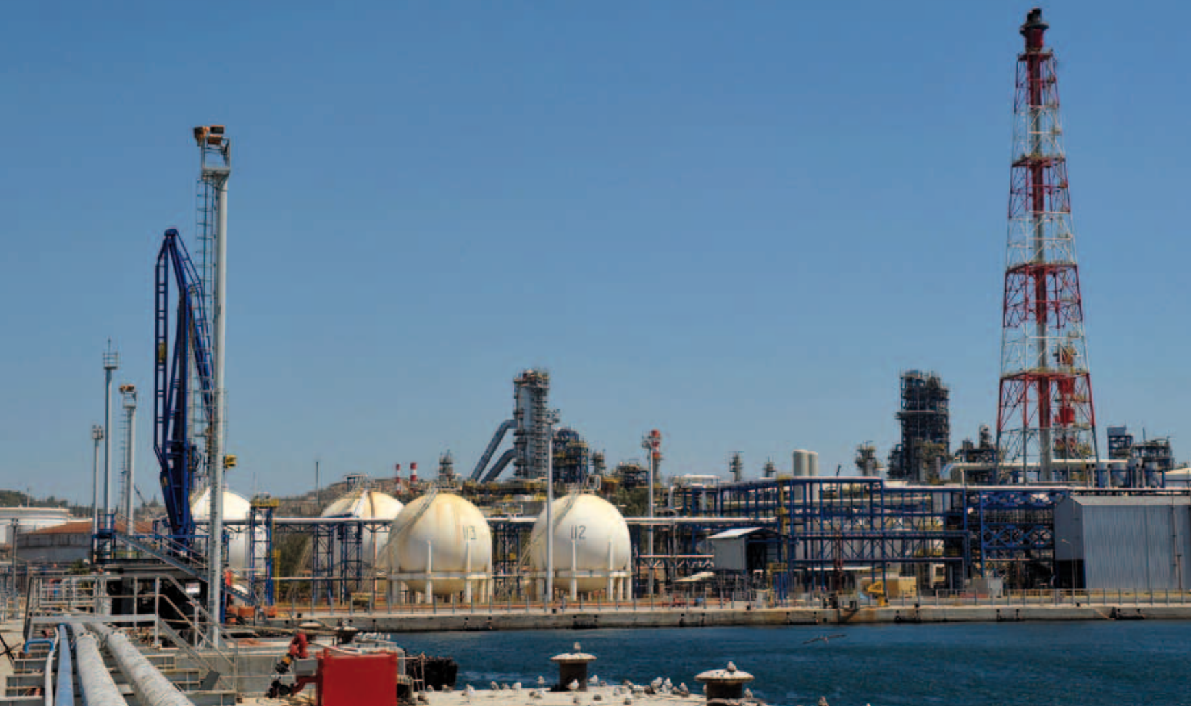
A View of Elefsina Industrial Installations
