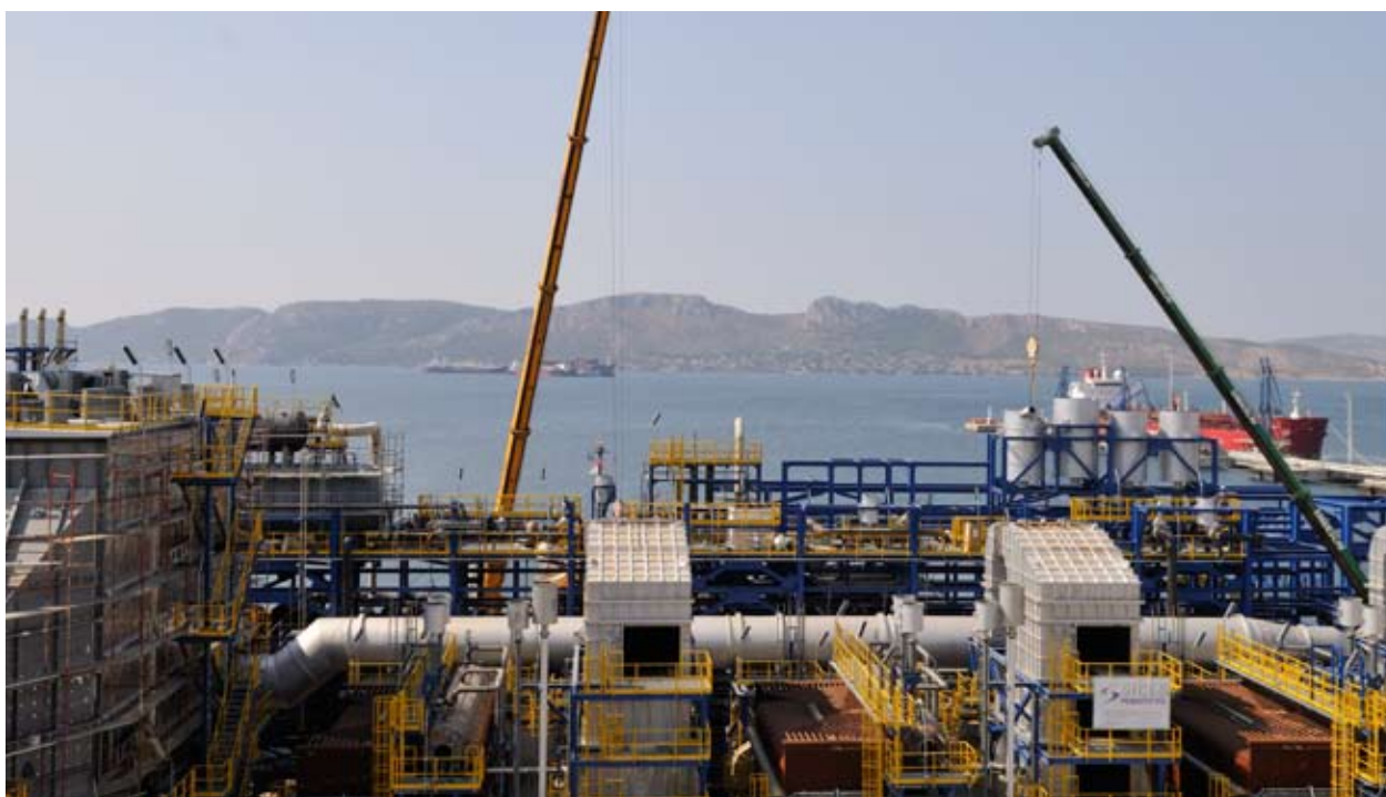
Upgrading Project at Elefsina Refinery
