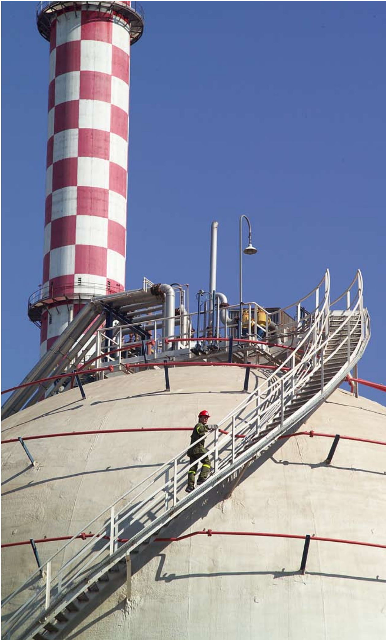
Products Storage Tank in BEA
