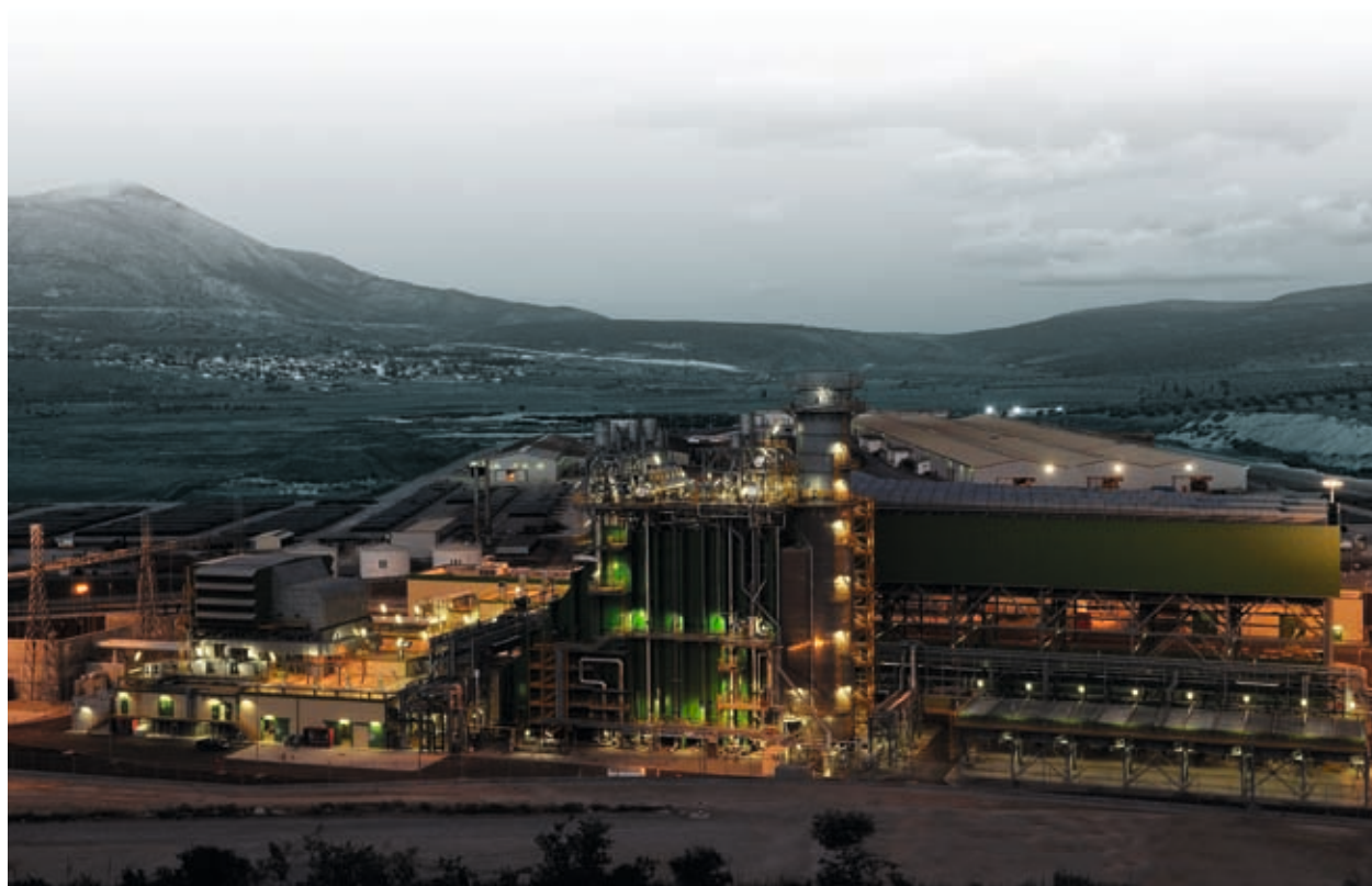
CCGT Power Plant in Thisvi
