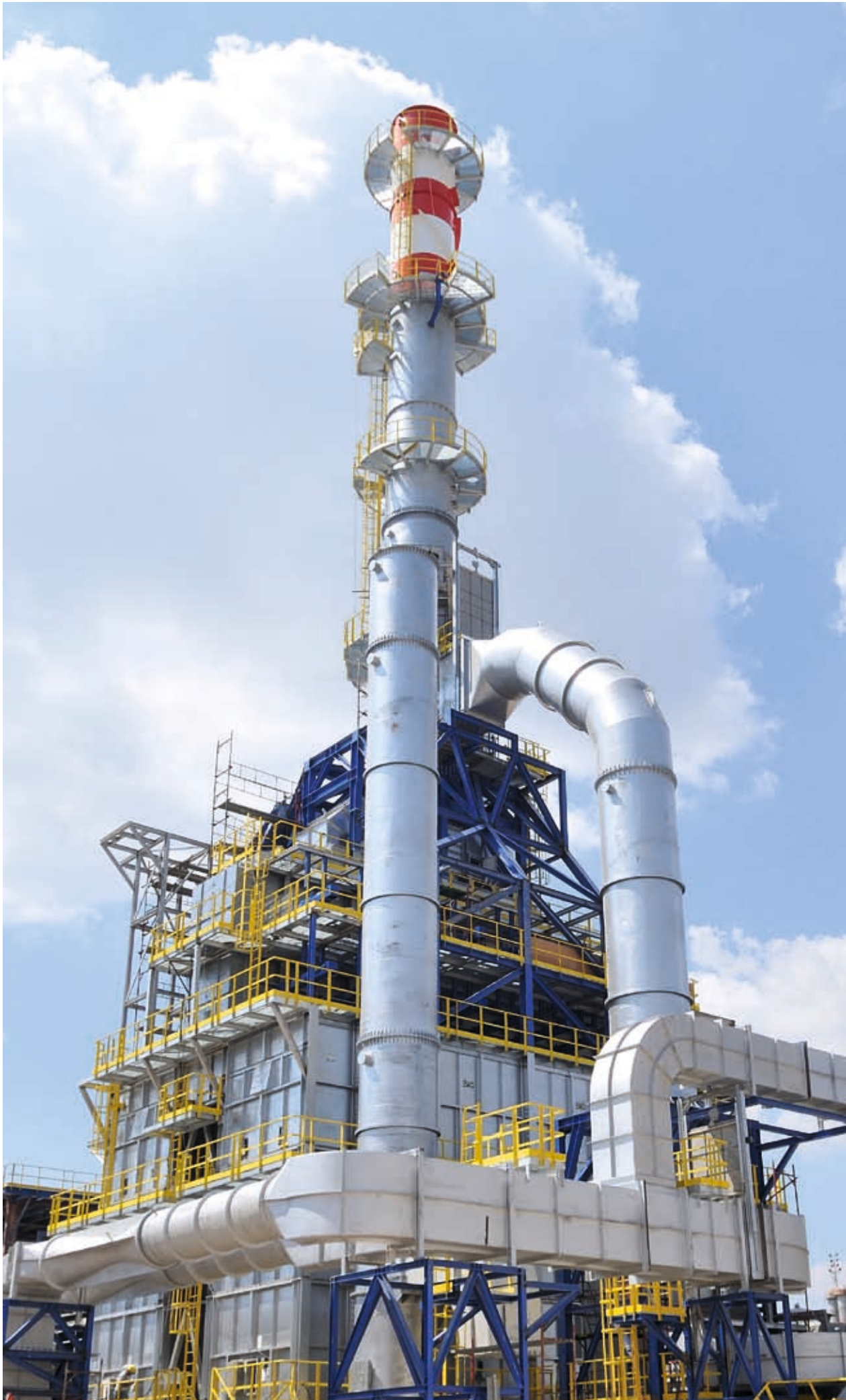
Upgrading project in the Elefsina Refinery
