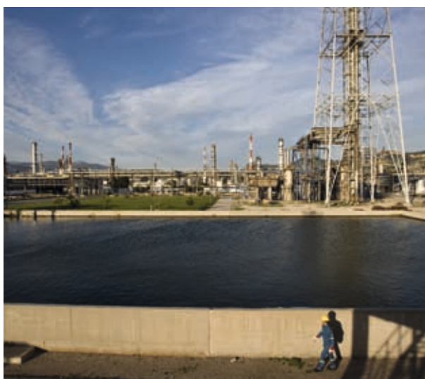
Firefighting lake in Aspropyrgos refinery
